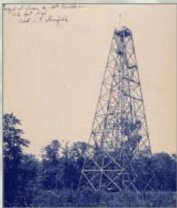
Typical tower for triangulation measurement
